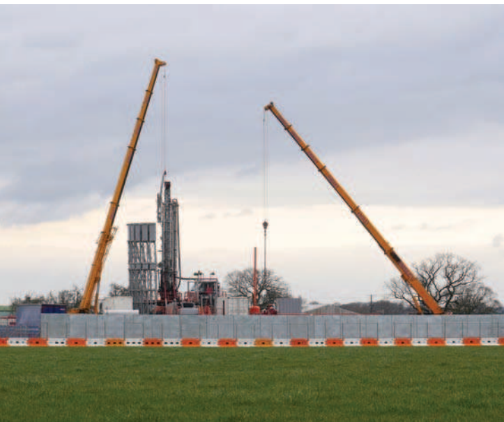
▲ Farndon, Chester. Dart Energy drilling CBM well in March 2014. (© Extreme Energy Initiative)
